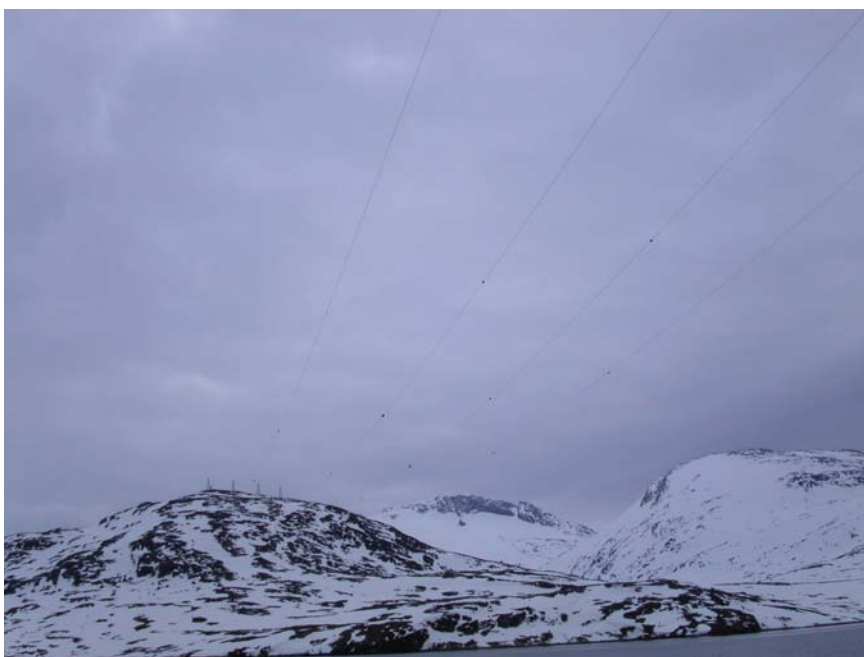
Difficult geography and supply security are expensive conditions. Transmission line Nuuk.
